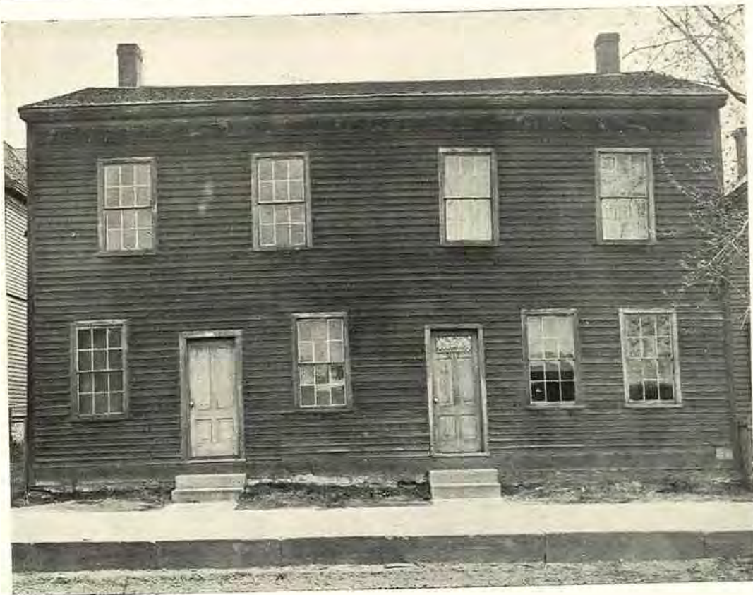
FIRST LODGE HALL USED BY CATARACT LODGE, MAIN ST. N. E., NEAR 4TH AVE.
